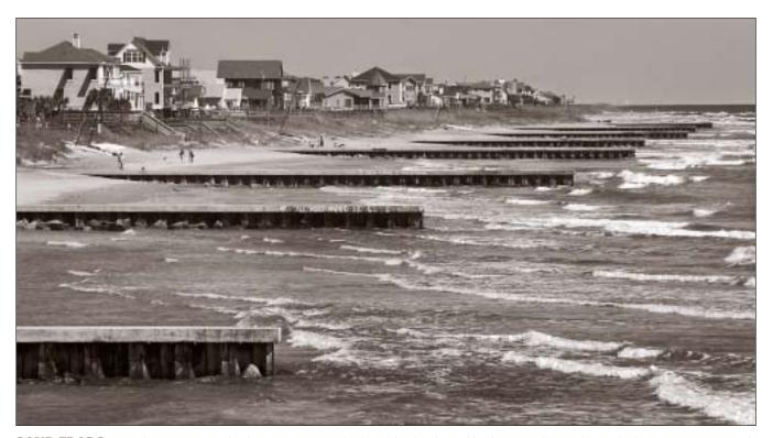
**SAND TRAPS.** Decades ago, groins—hard structures perpendicular to the shoreline—like these at Folly Beach were built in an effort to control erosion. Later, groins fell out of favor because they can starve sand from downdrift beaches. Now, under South Carolina regulations based on a recent state law, new groins can be constructed and existing groins can be reconstructed only in concert with an ongoing nourishment effort that meets special criteria. PHOTO/WADE SPEES
